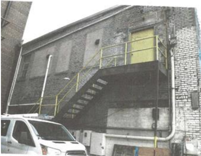
window replacement and repairs
