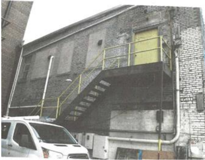
Before window replacement and repairs
